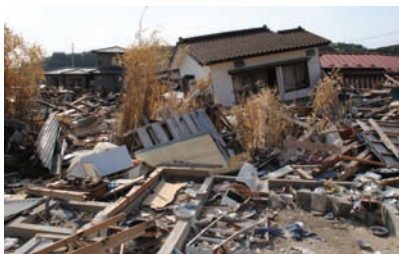
AN EXAMPLE OF THE TSUNAMI'S DESTRUCTION
